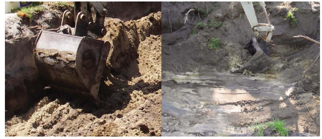
Fig. 1. Photos demonstrating rake method (left) versus scoop method (right) for excavation
