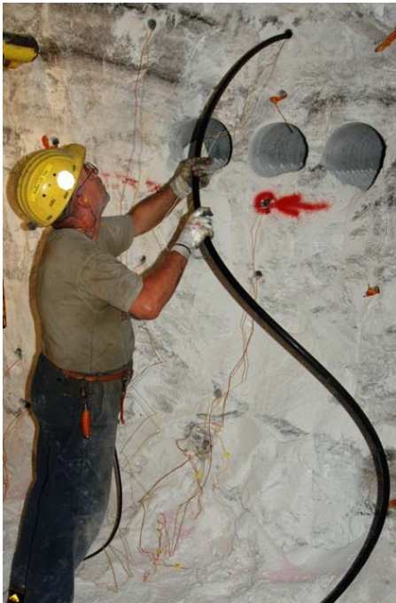
Adding explosive prior to blast
